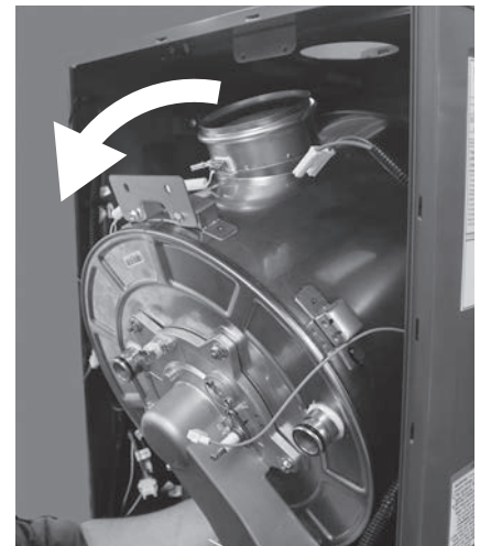
Figure 149 - Remove heat exchanger
